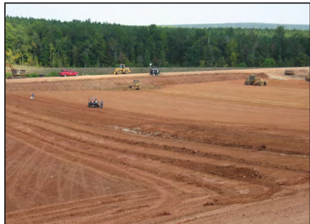
Phase IV Cells 3, 4 & 5 Construction
