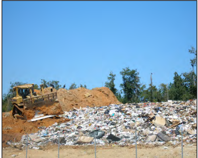
Waste Being Covered Daily
