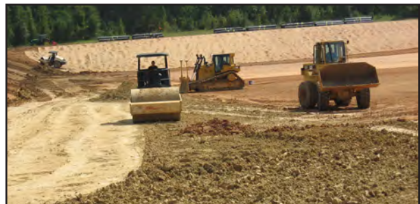
Installing Clay
