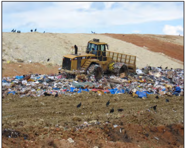
Compactor Working Waste
