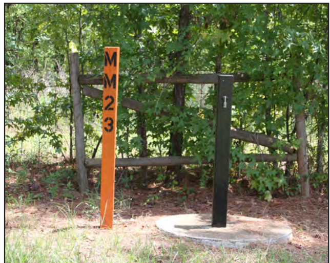
Methane Monitoring Well
