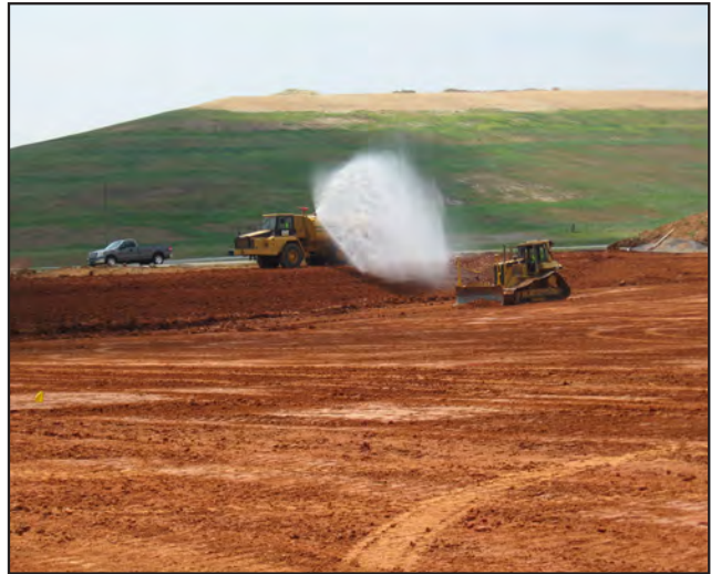
Applying Water To Clay Liner
