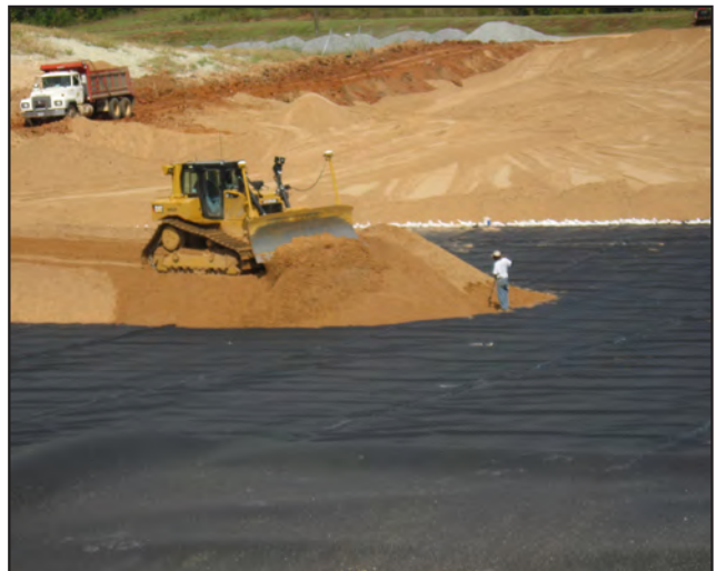
Placing Protective Cover
