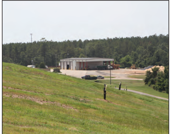
Well Field Phase II
