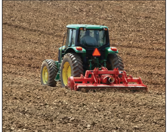
Processing Soil For Clay Liner
