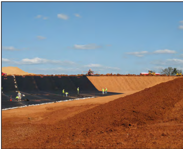
Liner Being Installed
